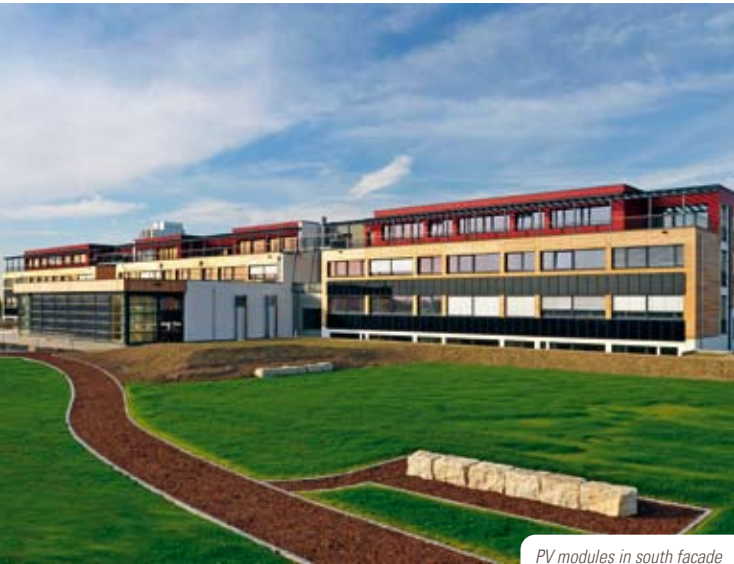
PV modules in south facade
